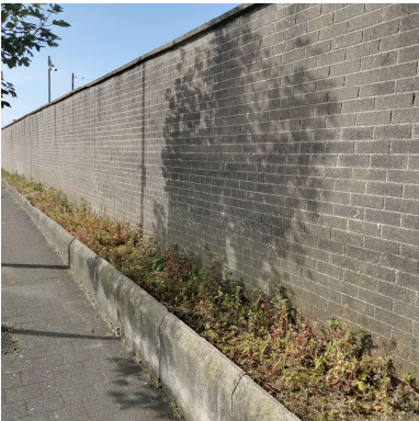
"Skip" wall at Community Centre
